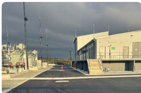
South Jerrabomberra build powers future growth.
